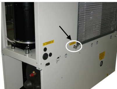
Fig. 3 Position of condensate drain
